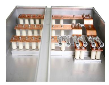
With the series flexible design and certification, we are able support up to 40 kV in zone 1/2, 21/22 and 1250 A.
