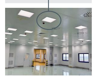
Our LED lighting portfolio includes floodlight, linear, tubolar, high / low bay and obstruction solutions as well as a recessed LED lamp which represents the right answer to the pharmaceutical industry's needs. Its housing is made of white painted steel sheet, stainless steel AISI304 and AISI316, ideal solution for clean rooms and it is fully compliant with ISO14644-1 for clean areas.
